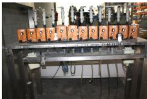
Reference: BPS-066 PUMP GROUP Year: . Brand: PROMINENT
