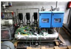
Reference: BPS-025 3 GROUP PUMPS WITH 2 GROUP UV ... Year: CRN 10-05 A-FGS-G-E-HQQE Brand: GRUNDFOS
