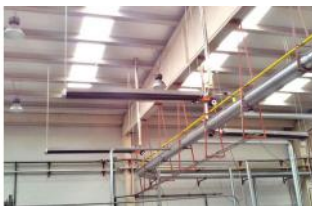
Reference: MOL-066 GAS HEATING RADIANT TUBE Year: . Brand: .
